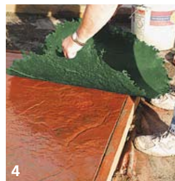
4 The patterned finish is created by placing the mats on the surface of the coloured concrete whilst it is still in its 'wet' state. The CCS stamping mats can also be used on fresh, integrally coloured concrete.
